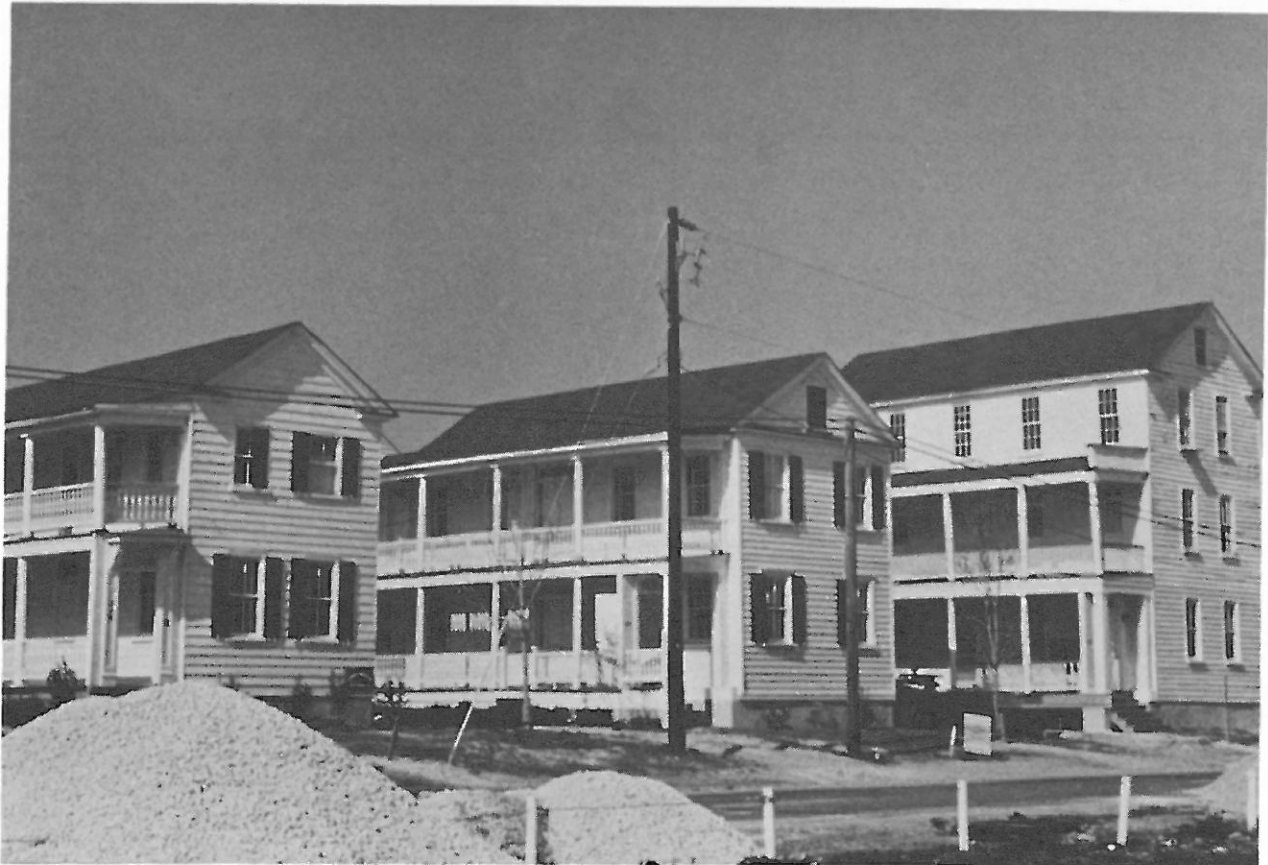
Figure 7a: The President Street site at the time of excavation, as seen from the University Services building.
